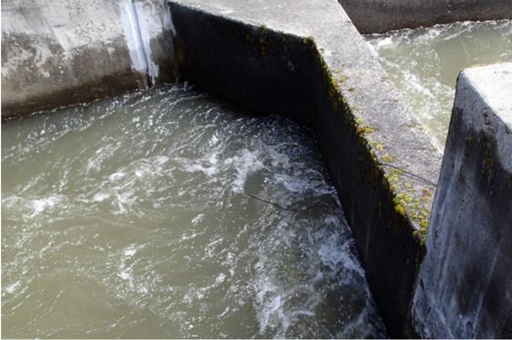
Figure 4. Deployed surface antenna.
