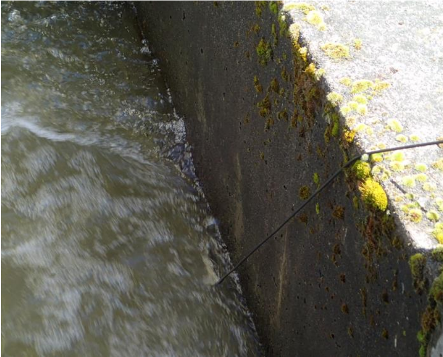
Figure 3. Deployed underwater antenna.
